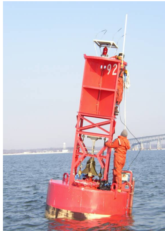
Woods Hole Group technicians installing a buoy-mounted current meter – Bay Bridge, Annapolis, MD
